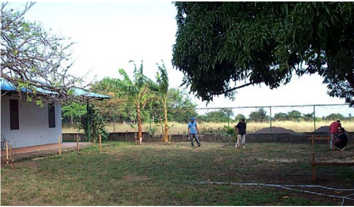
Just beginning – planning the foundation.
